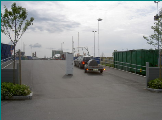
This plant for recycling of household wastes is built on a light weight construction made of fly ashes on clay soil
