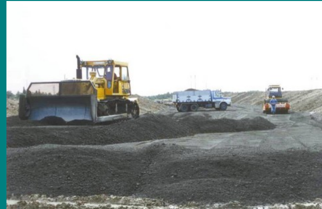
Lightweight motorway construction with grate bottom ash from coal-firing
