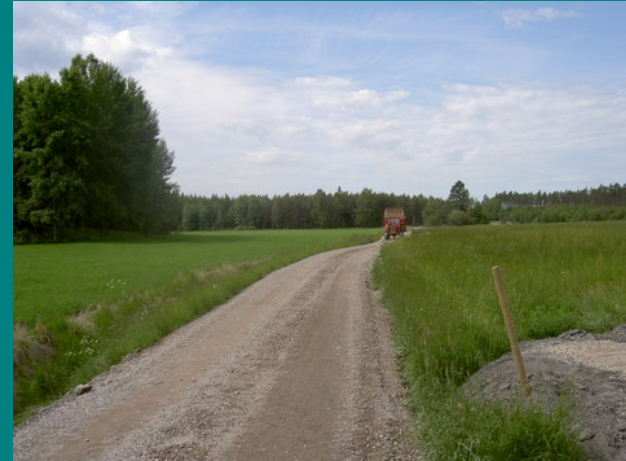
Fly ashes have transformed this to a very good road
